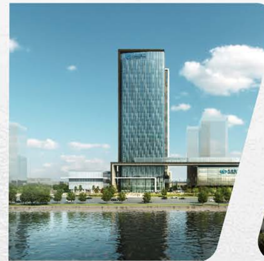
兴业银行大厦 Industrial Bank Building
