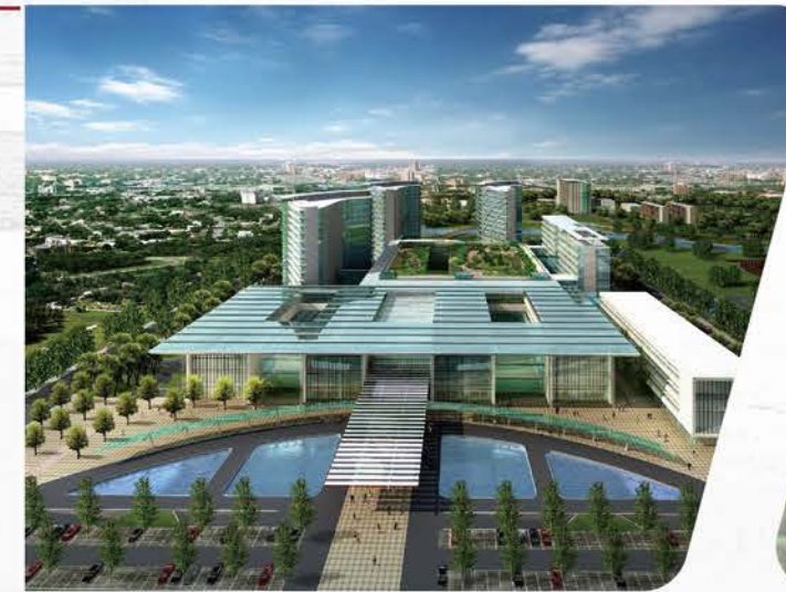
上海东方肝胆外科医院安亭院区工程 Shanghai Eastern Hepatobiliary Surgery Hospital Anting Branch Engineering
